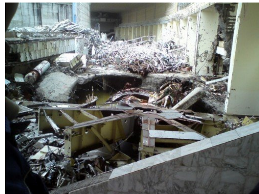
Figure 2. Engine room Sayano-Shushenskaya power plant before (left) and after (right) the accident ( www.lhp.rushydro.ru )
