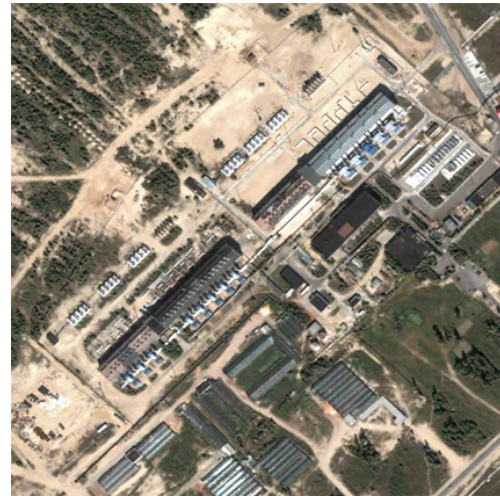
Figure 104. An image from Quick Bird satellite - gas-compression station
