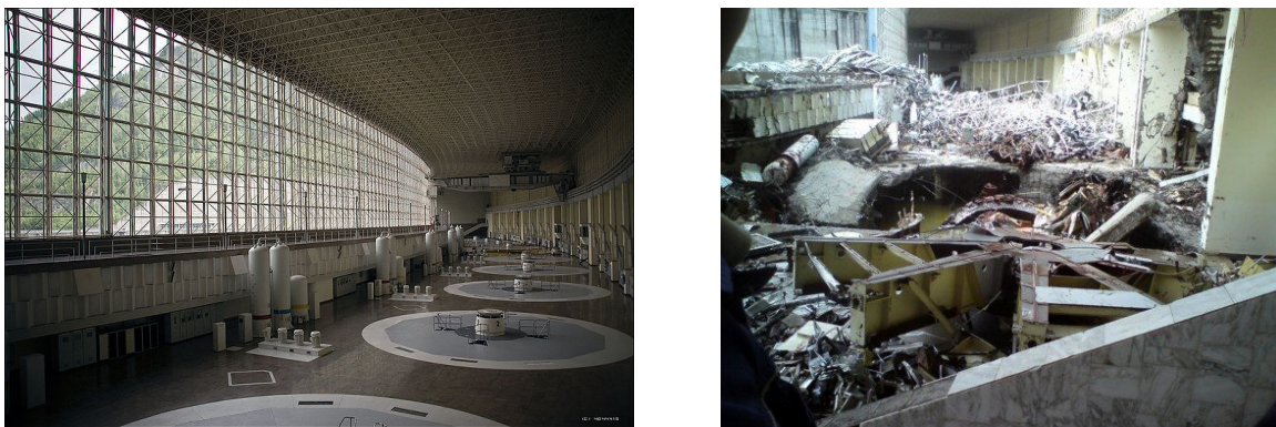
Figure 2. Engine room Sayano-Shushenskaya power plant before (left) and after (right) the accident ( www.lhp.rushydro.ru )
